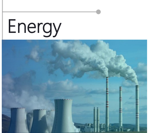
Oil, Gas, Power plants
