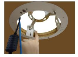
**NOTE:** The following illustration shows how the flush mount will look like when viewed from inside the ceiling. In case you cannot access inside the ceiling, use your fingers to position the retaining brackets through the hole.
